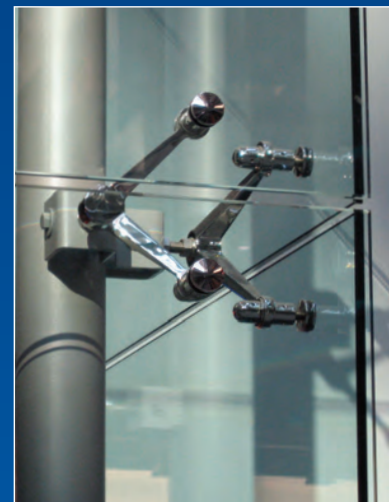
In a Glass Fin Supported System, vertical heavy glass fins are placed at 90 degrees to the glass wall. The Spider Fittings attach to both the fin and the glass wall.
